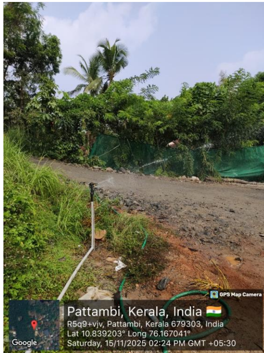
Figure 12: Photograph of water spraying on road
