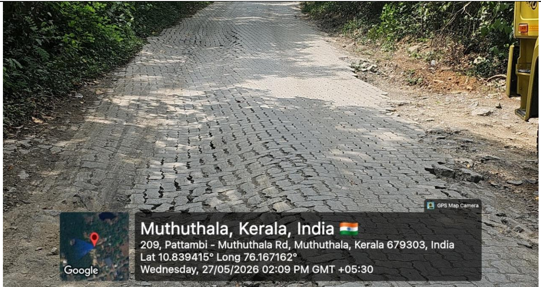
Figure 4: Haulage roads maintained with Inter locks
