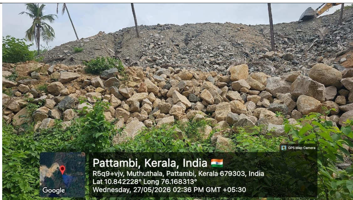
Figure 3: Ob dump heaped with gabion walls
